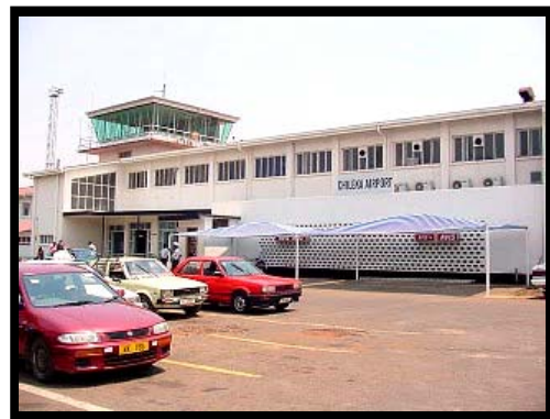
Chileka International Airport Blantyre, Malawi AFRICA
